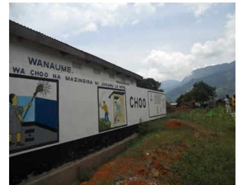
Toilet block requires water for flushing and washing.
