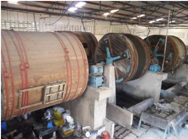
Tanneries for treating and manufacturing leather also require effluent treatment systems to avoid toxic chemicals from entering water.
